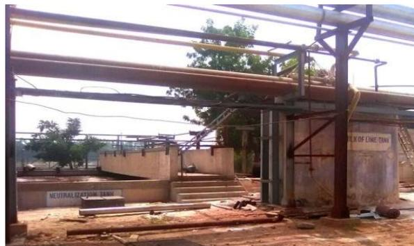
Fig. 2.7 Neutralization tank.
